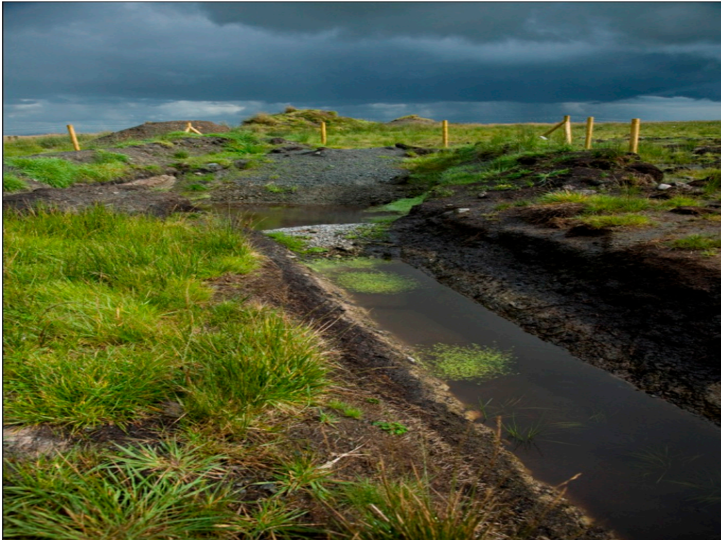
Figure 3-3: Swale draining to Settlement pond
