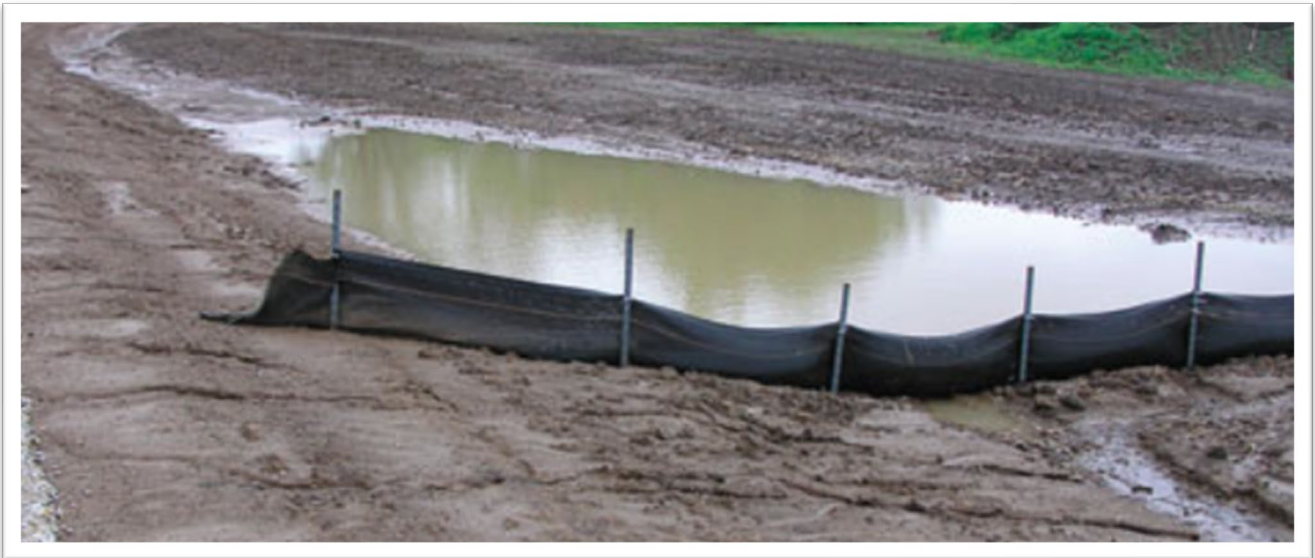
Figure 3-7: Silt Fence
