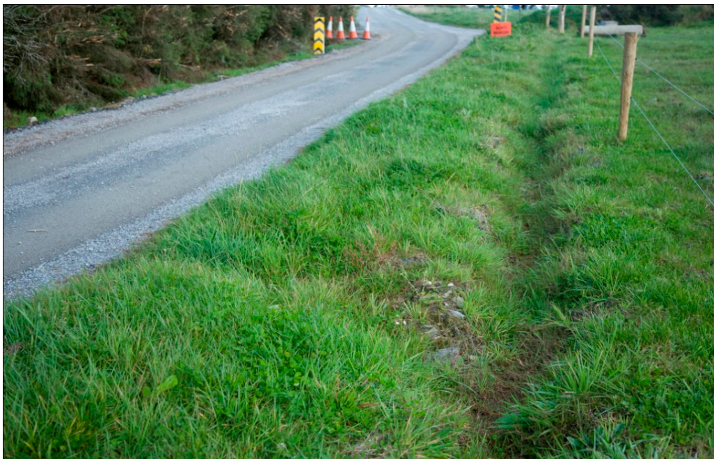
Figure 3-2: Grassed swale along access track
