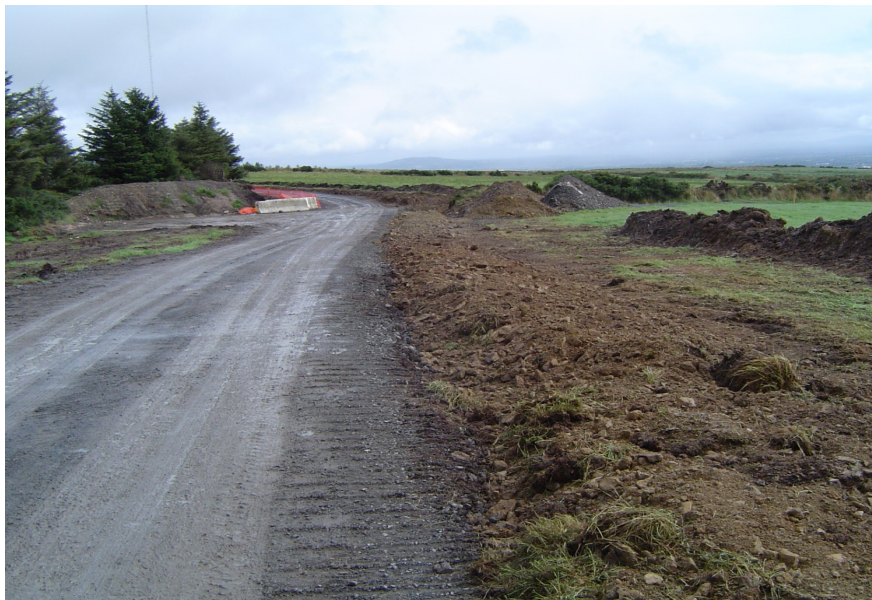
Figure 3-8: Backfill over cable trench
