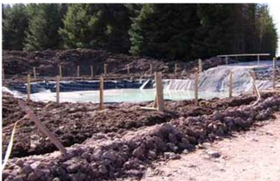
Figure 3-9: Lined Settlement Lagoon for Concrete Washout Facility
